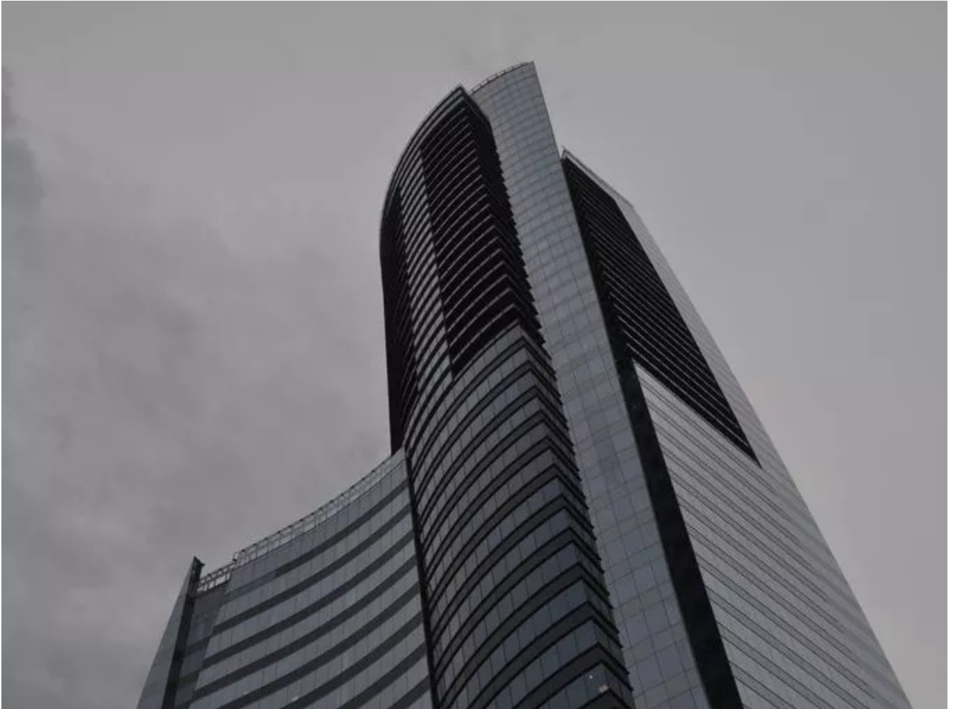
Buckhead's Sovereign tower. | Michael Kahn, Curbed Atlanta
